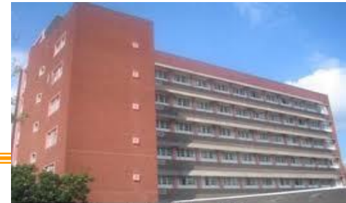
Renovated multi-story building
