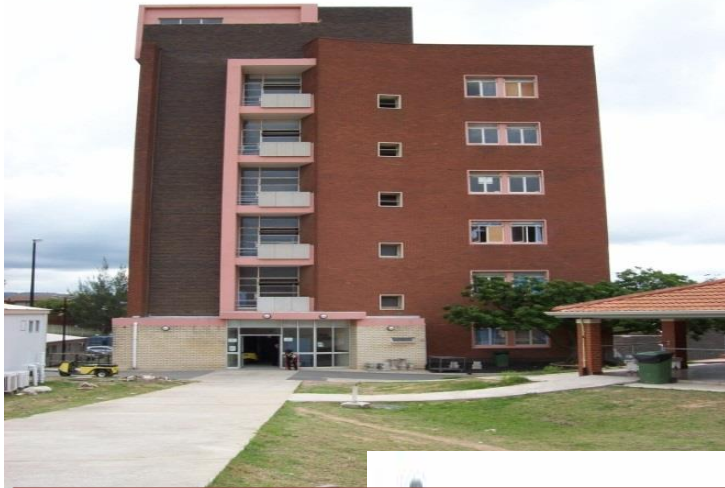
MDR Multistory Building
